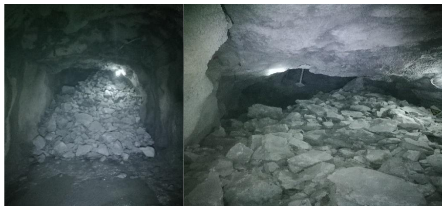
Figure 7. In situ stope blasting engineering effect.
