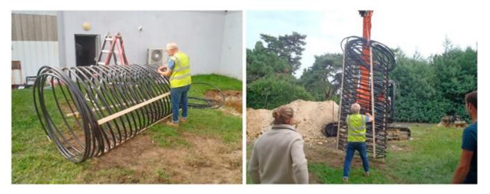
**Figure 1.** Installation of a spiral (earth basket) ground heat exchanger with a fibre-optic distributed temperature sensing system at the IUT Civil Engineering Student Laboratory (Bordeaux, France) pilot site (picture: Groenholland Geo Energy systems).
