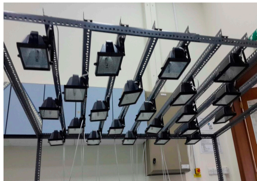
Figure 5. Solar simulator used in tests.
