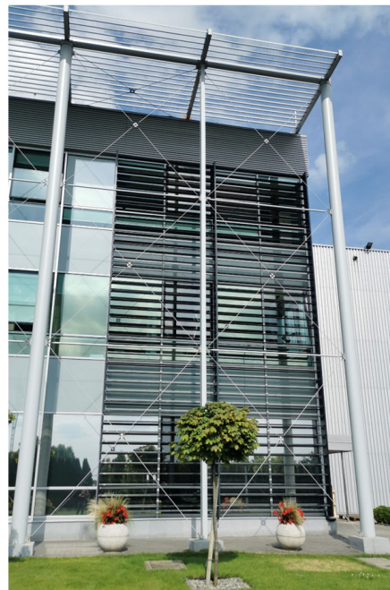
Figure 1. Real view of dynamic building façade with PPV panels.
