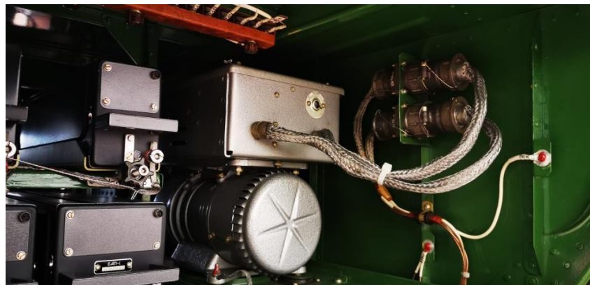
Figure 2. Installation of the PT-125C inverter.
