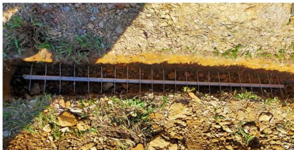
Figure 3. Installation of the linear array ground electrode in the trench.
