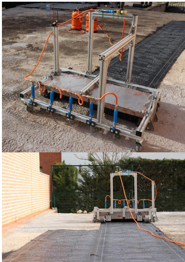
Figure 18. Asphalt rolls installation results.
