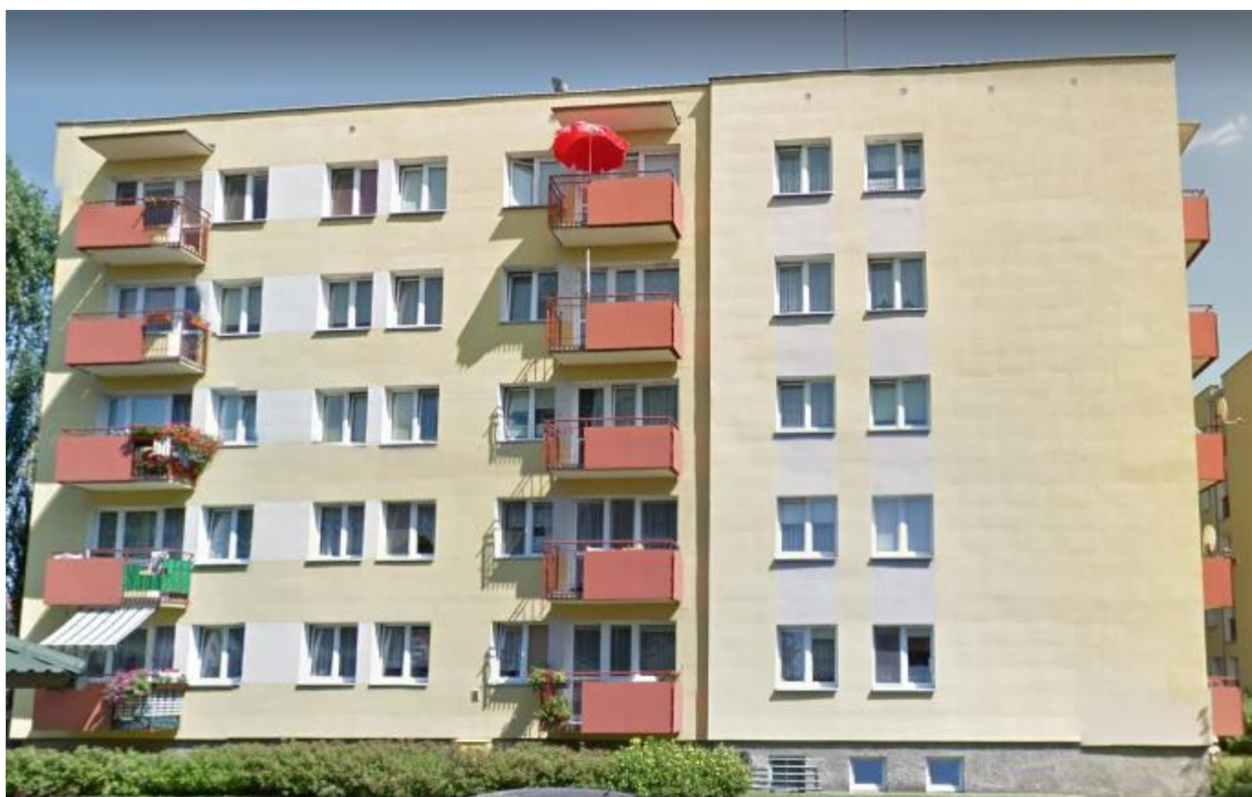
Figure 6. View of the analysed multi-family building.
