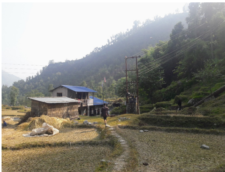
Figure 2. The MHP powerhouse in Salyan, the case study community.
