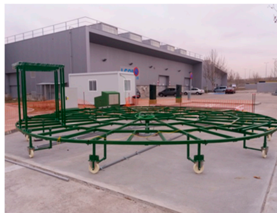
Figure 19. Image of platform base construction with rectangular profile of 60 \times 40 mm.
