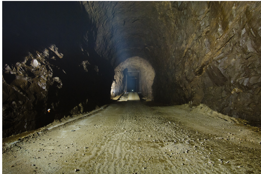
Figure 3. Picture of a prototype sand trap tunnel at hydropower plant; courtesy of Sira-Kvina kraftselskap.
