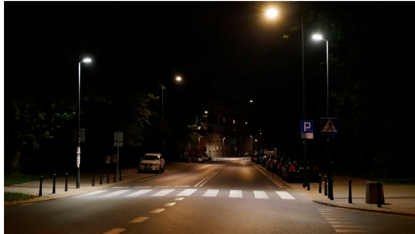
Figure 7. View of a representative section, Section 24.
