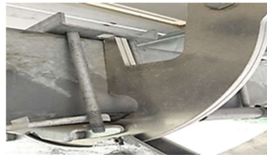
Figure 9. New pile head installed at a tracker.
