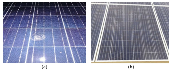
Figure 8. (a) Damaged solar PV module and (b) damaged module replaced with a new one.
