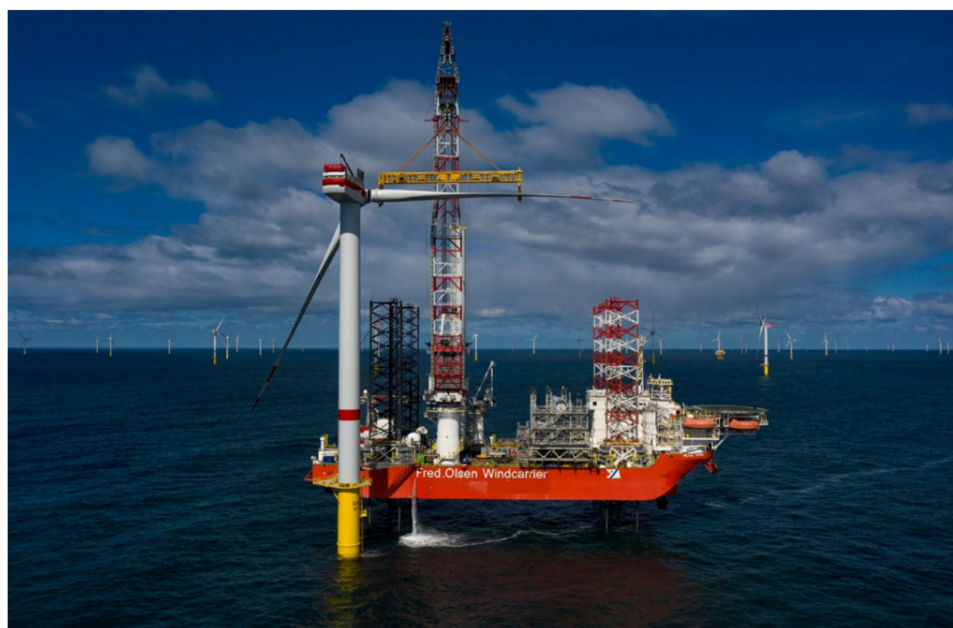
Figure 2. Blade installation taking place at Trianel Windpark Borkum II.
