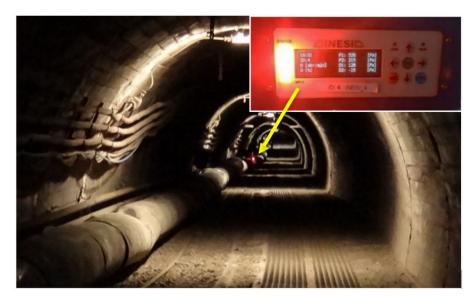
Figure 15. Response of the measuring module for the connector unsealing (red light).
