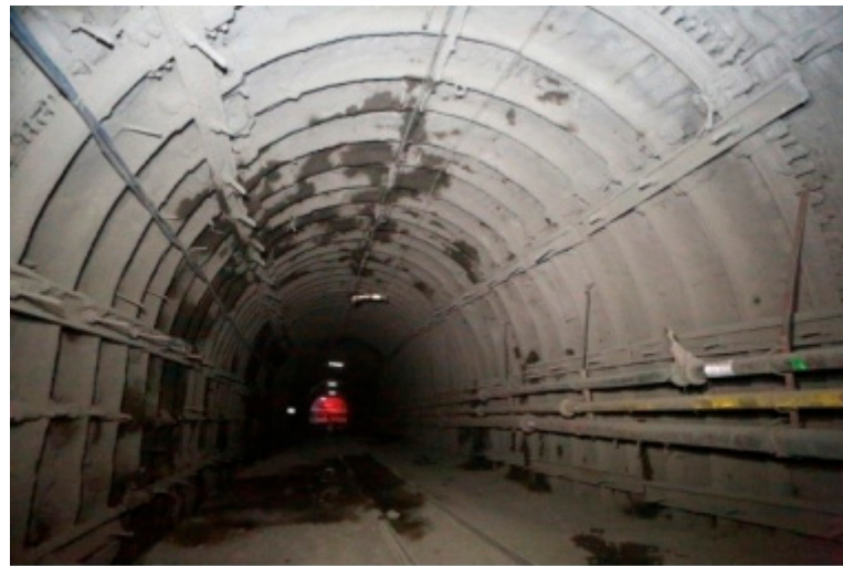
Figure 16. Tested support scheme.
