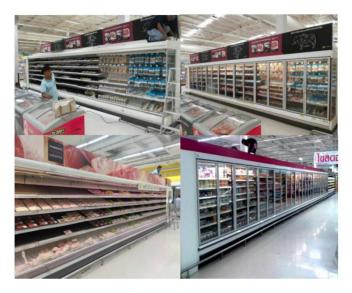
Figure 2. Installation of Low-E glass door for store No.1 (R22).
