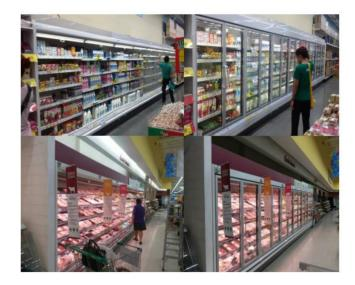
Figure 3. Installation of low-E glass door for store No.2 (R404A).
