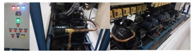
Figure 4. Digital compressor rack with digital compressor and digital controller No.1 (R22).
