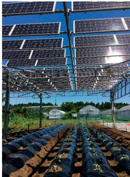
Figure 2. Photo of agrivoltaic system (from Yajima et al. [50]).
