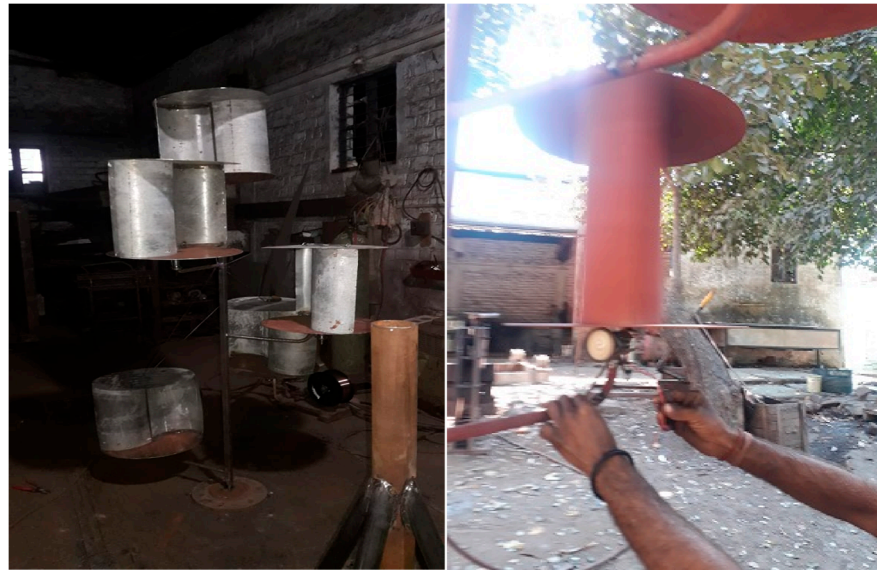
Figure 7. Fabrication of the Savonius wind tree.
