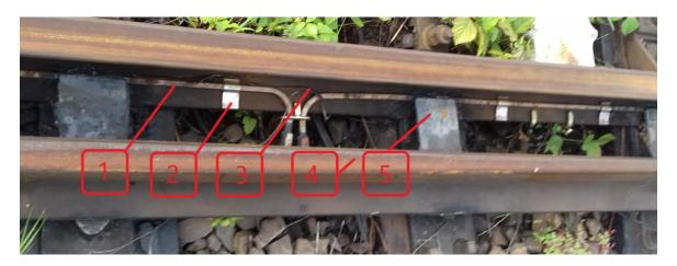
**Figure 2.** Built-in flat-oval resistance heaters (1) mounted with special holders (2) to the foot of the stock rail (3); (4)—switch rail, (5)—plates.
