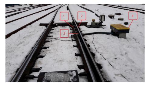
**Figure 1.** Built-in elements of the turnout electric heating system (1—switch rail, 2—stock rail, 3—working space, 4—separation transformer boxes).
