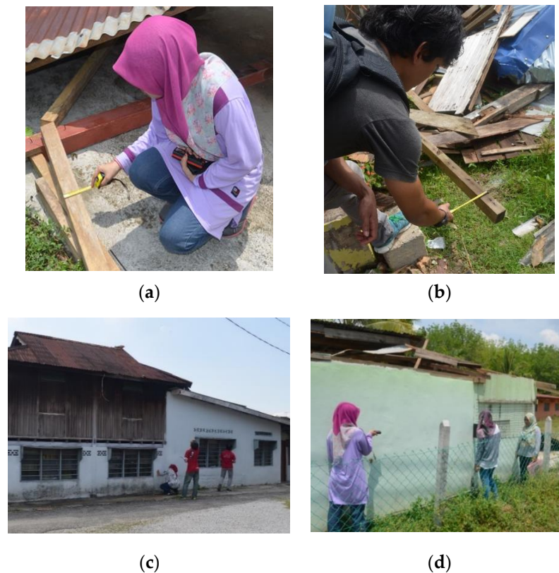
Figure 3. Measurements of the (a) roof truss width; (b) roof truss thickness; (c) height of the house; and (d) width of the house.
