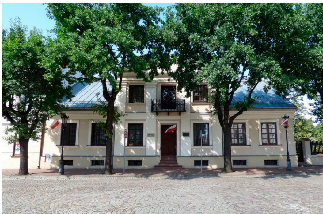
Figure 1. The renovated building.
