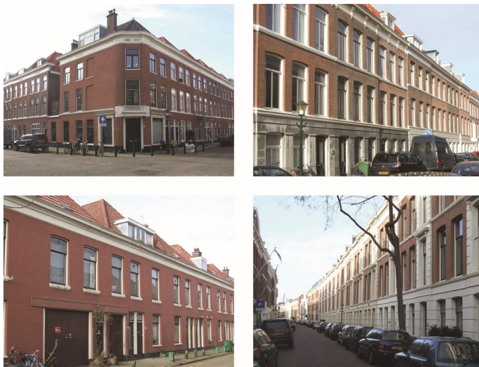
Figure 4. Residential buildings are usually in eclectic style with a variation in size. The brickwork architecture is sometimes simple, sometimes detailed. Photographer: Leo Oorschot.
