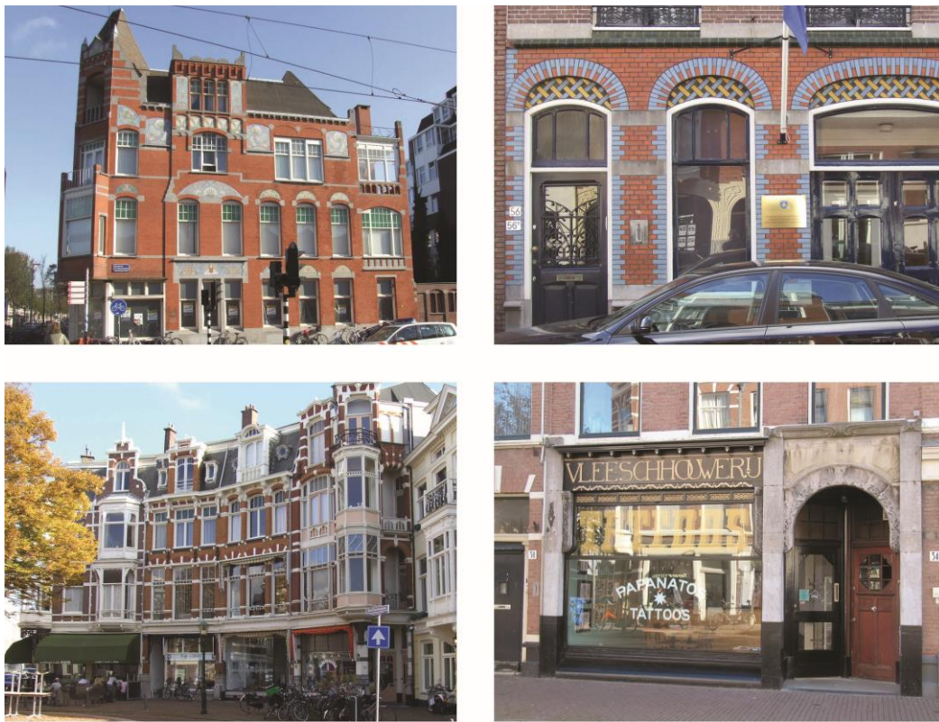
Figure 5. Public buildings are usually in Dutch neo-renaissance, and shops in beautifully designed fin de siècle architecture. Photographer: Leo Oorschot.
