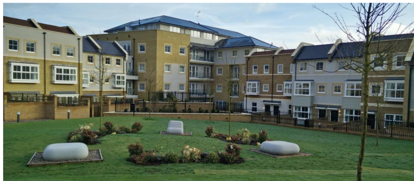
Figure 1. View of the housing development from the courtyard.
