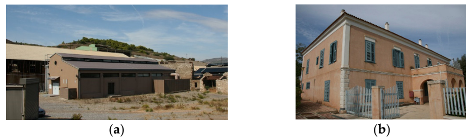
Figure 5. Testing boundaries of LTCP: (a) Building #1—H2 (active); (b) Building #2—admin (passive).
