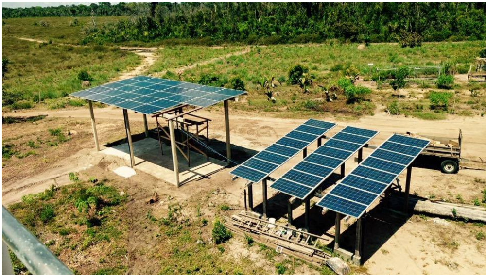
Figure 6. Installation of modules added to the hybrid system.
