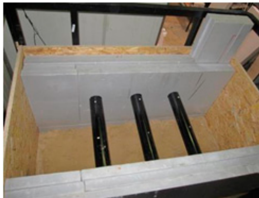
Figure 2. Placement of power cables in the sand.
