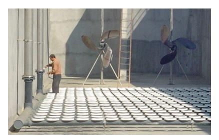
Figure 1. Fixed bottom aeration grid and agitators [5].
