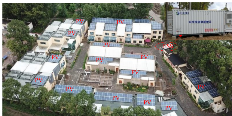
Figure 18. The vertical view of the microgrid system.
