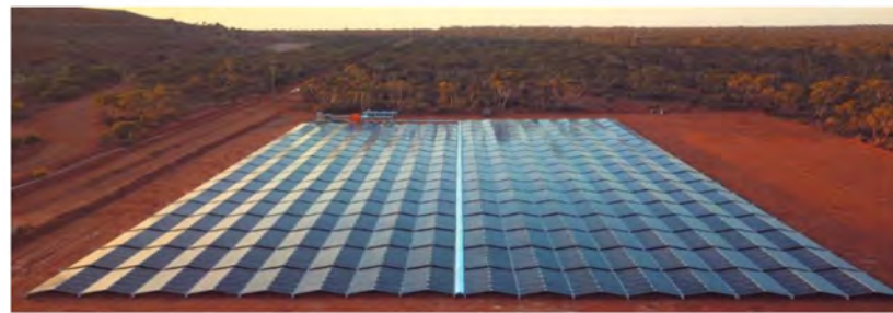
Figure 4. A ground mounted 1 MW system (Nomadic Energy, Western Australia). Reprinted with permission from [27]. Copyright 5B Australia Pty Ltd., 2021.
