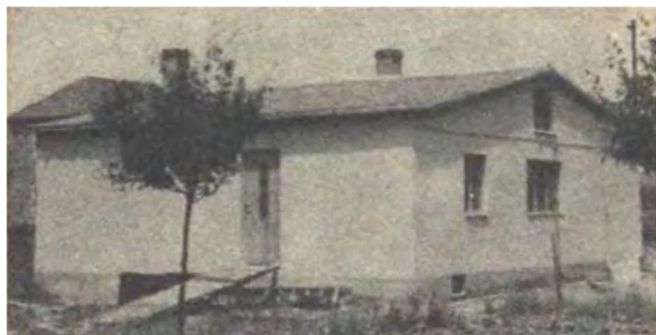
Figure 3. A family house made of SOLOMIT boards, a product of the company OSP Olomouc, Czechoslovakia (1959) [44].
