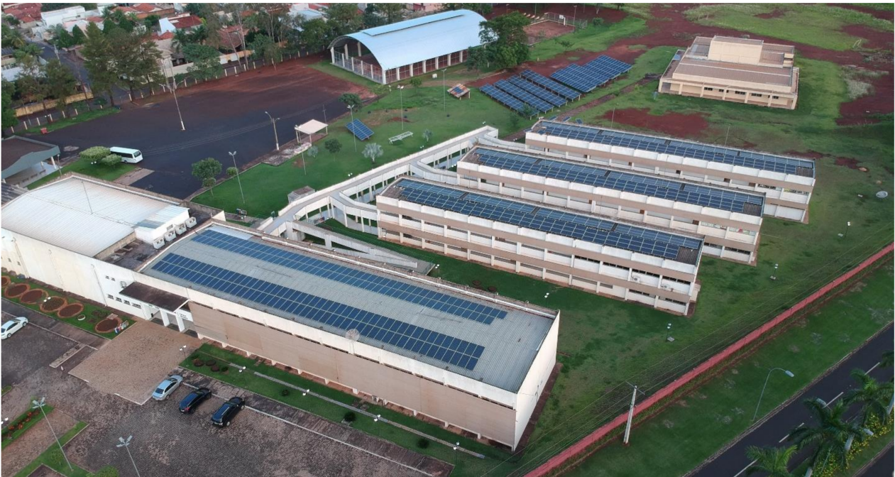
Figure 7. PV System—Itumbiara Campus.
