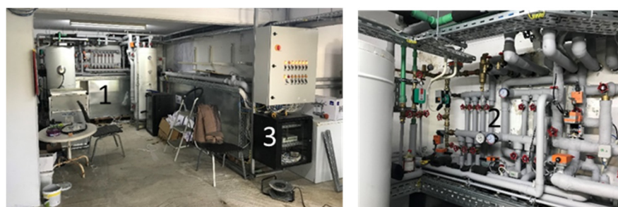
1 - TES Tanks; 2 - Control System Box; 3 - Water circuits and manifolds
