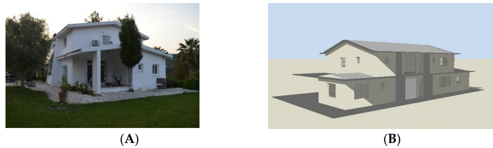
Figure 3. External view of the building—East. (A) = actual building, (B) = geometric model.
