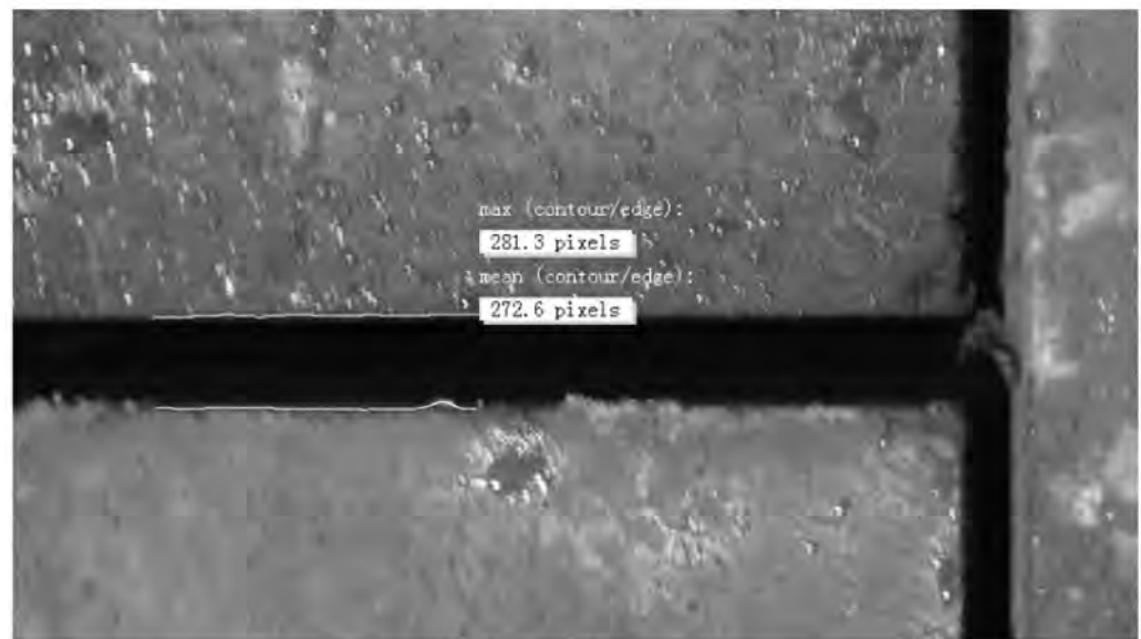
Figure 18. Segment joint width identification.
