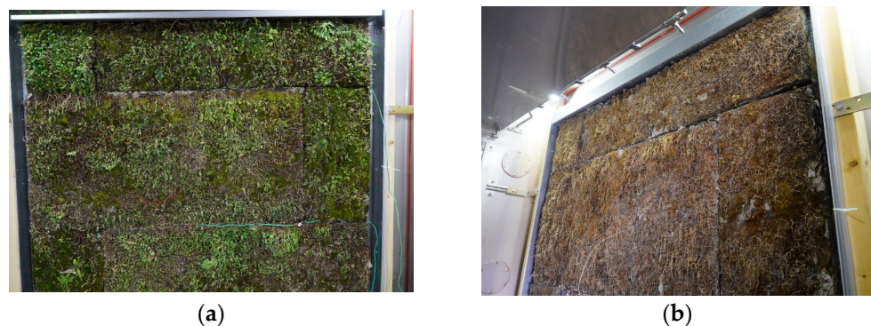
Figure 2. View of the outer skin before (a) and after the measurement (b). Despite heavy watering at the end, the vegetation was very dry, which was caused by the simulated solar radiation (simulated steady-state test, which is not presented in this paper) and water pump failure.
