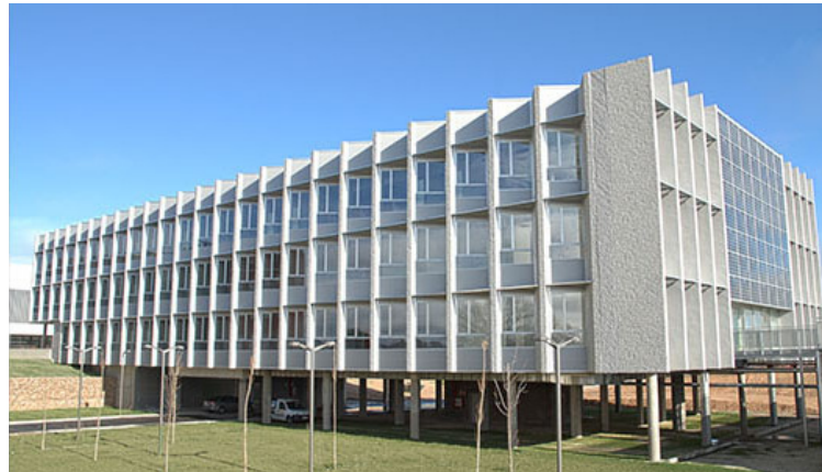
Figure 1. General view of the LUCIA building.
