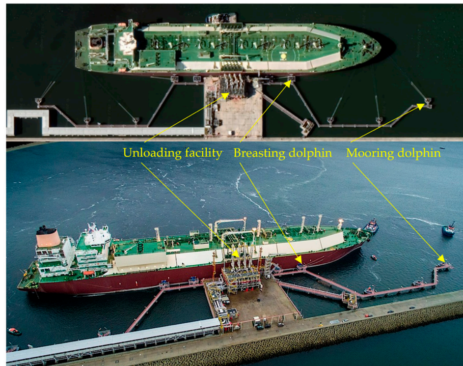
Figure 10. Unloading jetty and LNG carrier (based on [45]).
