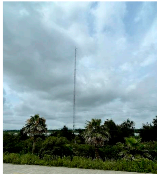
Figure 3. Wind measuring tower.
