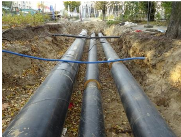
Figure 1. Example of pre-insulated heating pipes located in the ground layer at a depth of up to 1 m.
