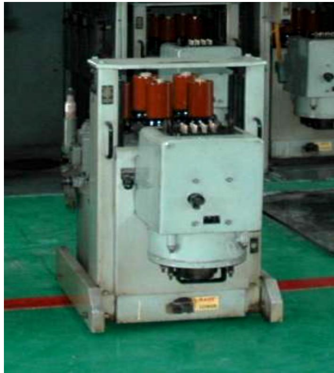
Figure 4. Sample of bulk/minimum oil circuit breaker [13].
