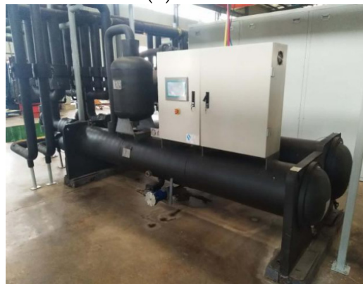
(c) Water source heat pump
