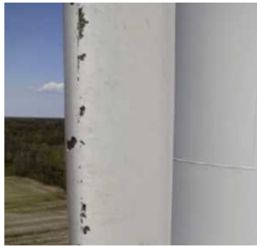
Figure 2. Photo of the leading edge erosion [29].
