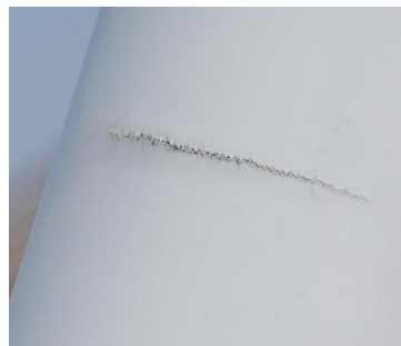
Figure 3. Photo of the micro-cracking on the blade [30].
