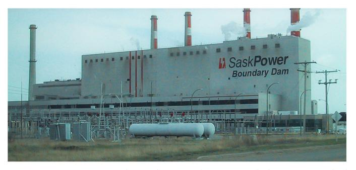
**Figure 3.** SaskPower carbon capture and storage project, Saskatchewan province, Canada. This project involves post-combustion capture of CO<sub>2</sub> accompanied with CO<sub>2</sub>-EOR [65].
