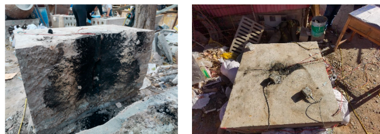
Figure 5. The test block after blasting.
