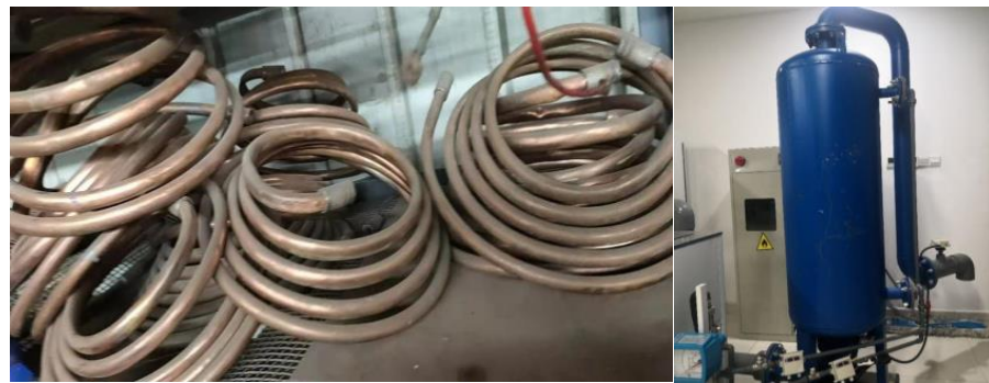
Figure 2. Internal copper tube and external integral structure of single spiral-tube heat exchanger.
