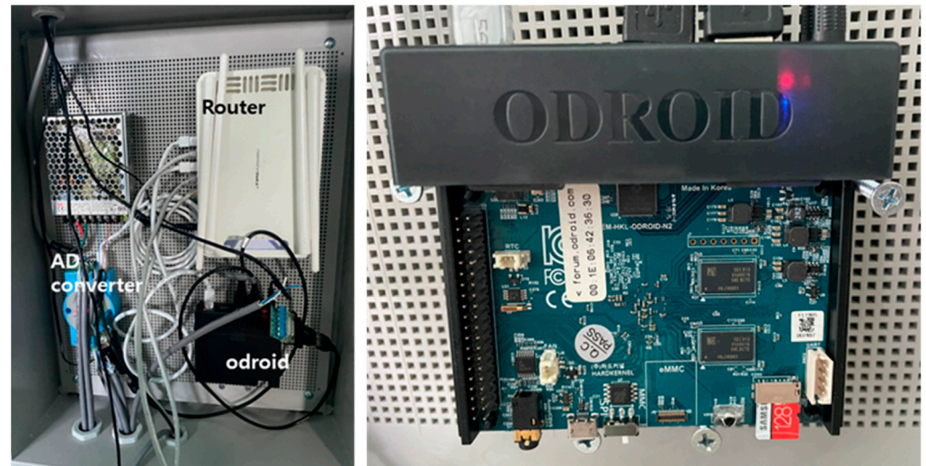
Figure 3. Monitoring devices installed on site.
