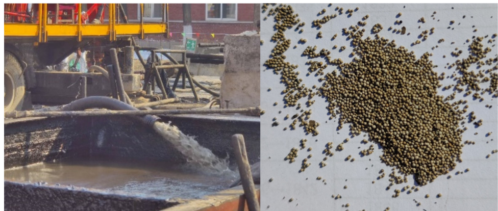
Figure 23. Returning fluid and sand output during the flushing process.
