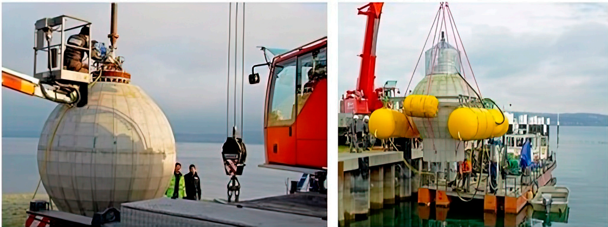
Figure 7. Lake Constance offshore pumped storage experiment in 2017 [53].
