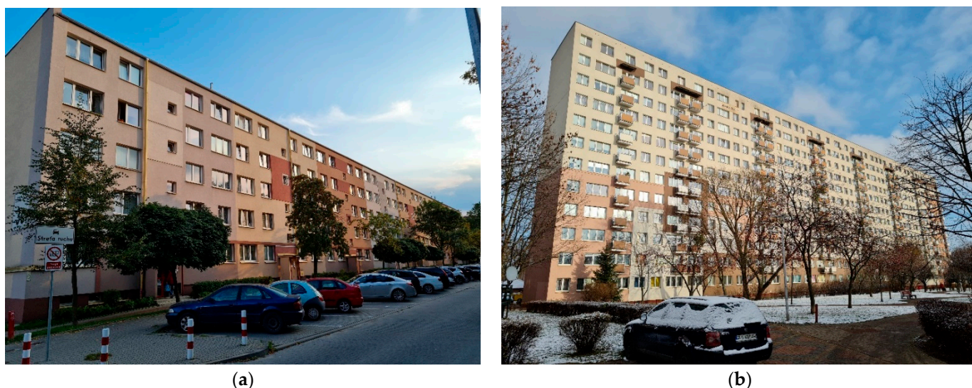
Figure 7. Prefabricated buildings in the "large-panel system" OW-T/67 style: (a) a 5-storey building, the most common in Poland, 3 Piastowska St., the first to be built in Białystok in 1969; (b) an 11-storey building, 11 Mieszka I St., shown in 2021, source: authors—photo A. Turecki.
