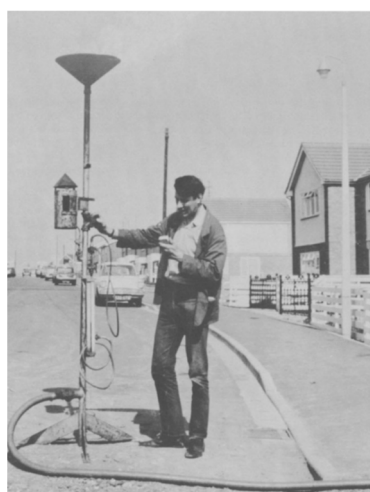
Figure 5. Town-gas-to-natural-gas transition field work in a Midlands town in England [50].
